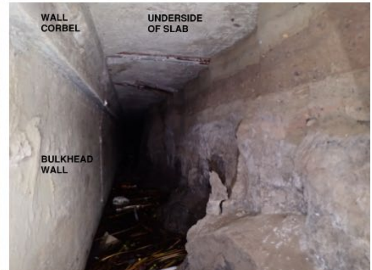
VOID LOOKING EAST FROM SLAB OPENING
