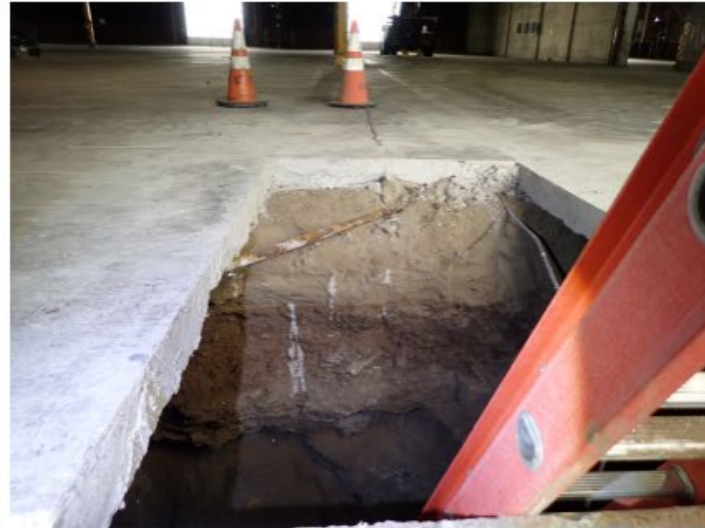
FILL AND SOIL LAYERS AT SLAB OPENING
