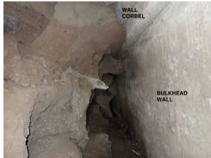
VOID LOOKING WEST FROM SLAB OPENING
