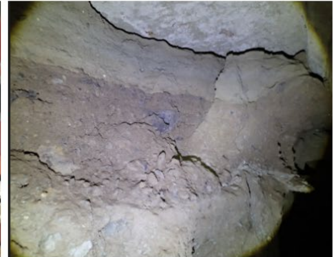
FILL AND SOIL LAYERS AT SLAB OPENING
