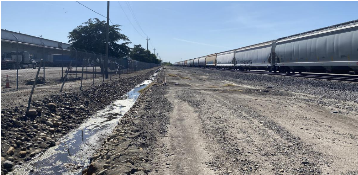
Figure 2: Existing Ditch along McCloy Avenue
